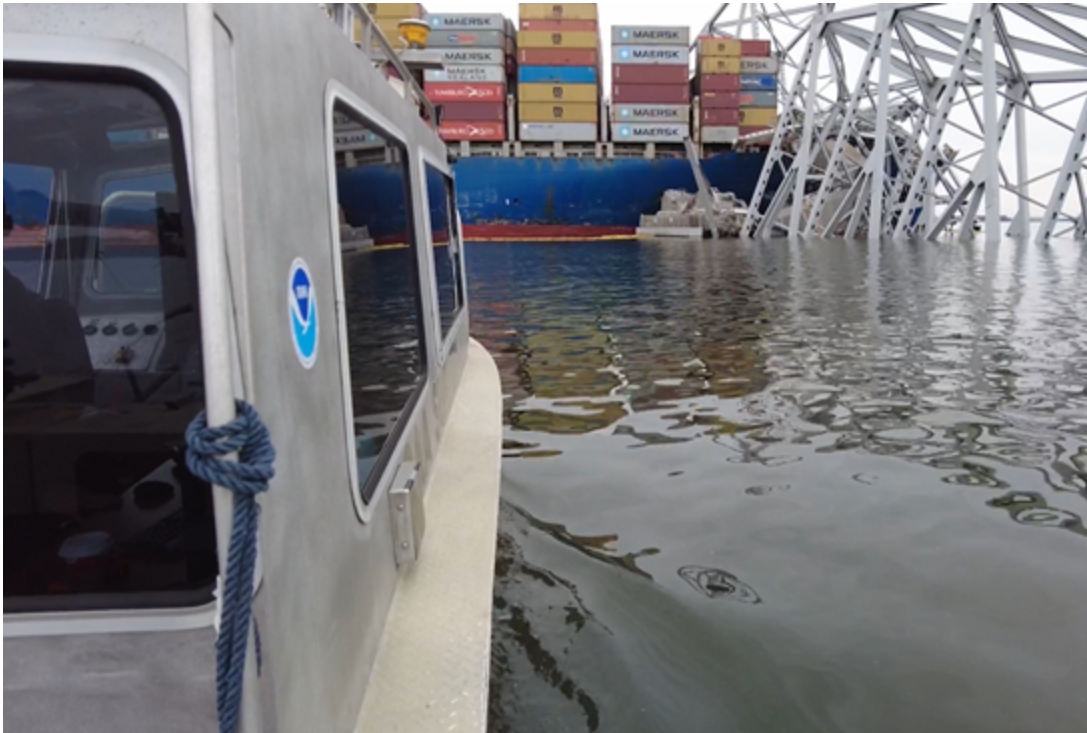
Figure 2: NOAA's navigation response team surveying close to the Dali after impact with the Francis Scott Key Bridge to identify temporary auxiliary channels and locate debris from the wreckage (NOAA/Bob Schwartz)
