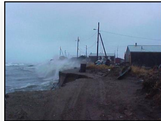
Photo 10: Shoreline erosion during coastal storm in Shismaref. (Credit: Tony Weyiouanna)
