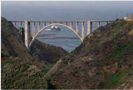
Bixby Bridge, Big Sur, California Photo Credit: CA Dept of Water Resources
