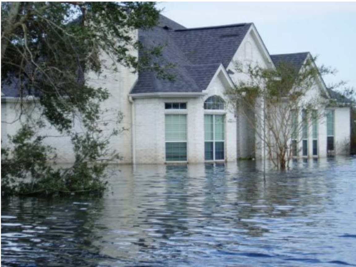
Flooding caused by Hurricane Ike in LaBelle, Texas. This house has since been demolished. Photo courtesy of Caroline Miller.
