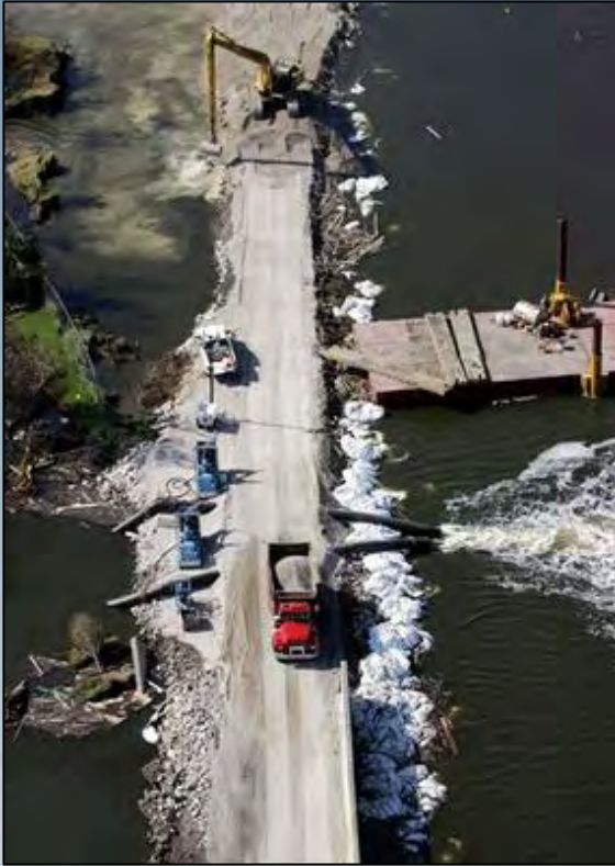
17 th Street Canal Breach
