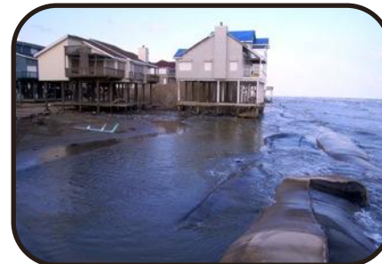
Flooding & Storm Surge
