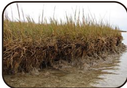
Bay Shoreline Erosion
