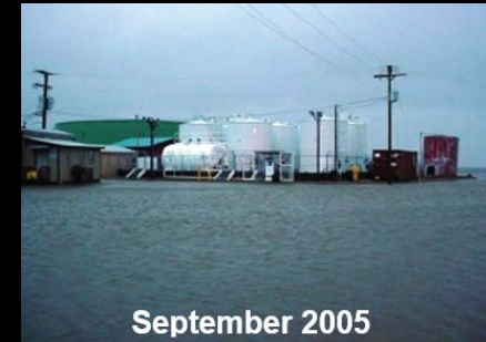
Fuel tanks flooded or at risk from erosion
