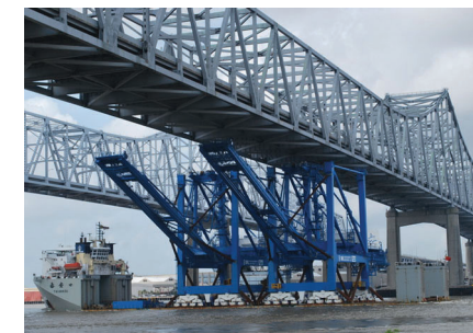
Cranes use PORTS® air gap information while passing under the Crescent City Bridge in New Orleans, Louisiana. Credit: Port of New Orleans
