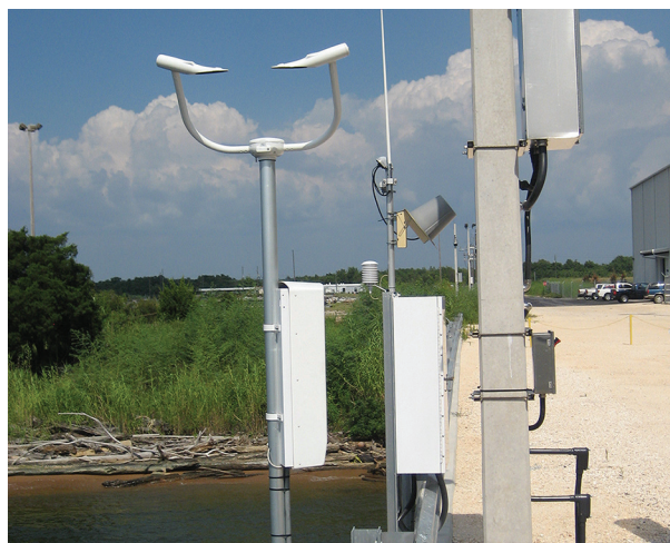
Visibility sensor at Pinto Island on Mobile Bay is primarily used to determine fog on the waterway. Credit: CO-OPS
