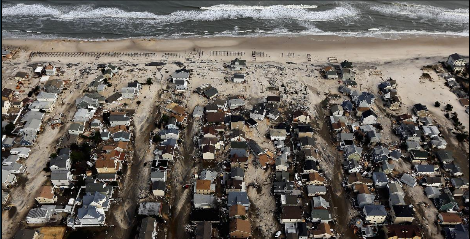
Seaside Heights, NJ after Hurricane Sandy (2012)
