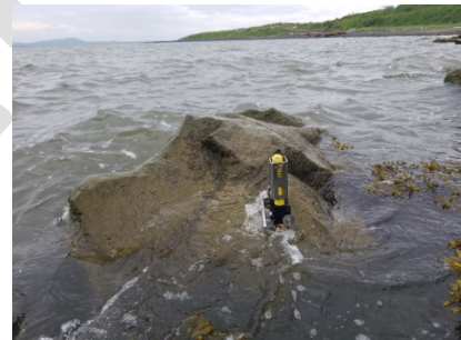
Figure 10. RBR Solo Depth Logger installed at St. Michael, Alaska. This is a non-vented pressure sensor that was intentionally installed above MLLW to measure a portion of the tide range.
