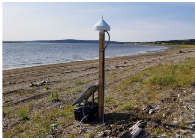
Figure 12. GNSS-Reflectometry water level system installed in Koyuk, AK by JOA Surveys, LLC in support of the NOAA Office of Coast Survey Project OPR-R385-KR-20. TerraSond Ltd. was the prime contractor. Photo courtesy of JOA Surveys.
