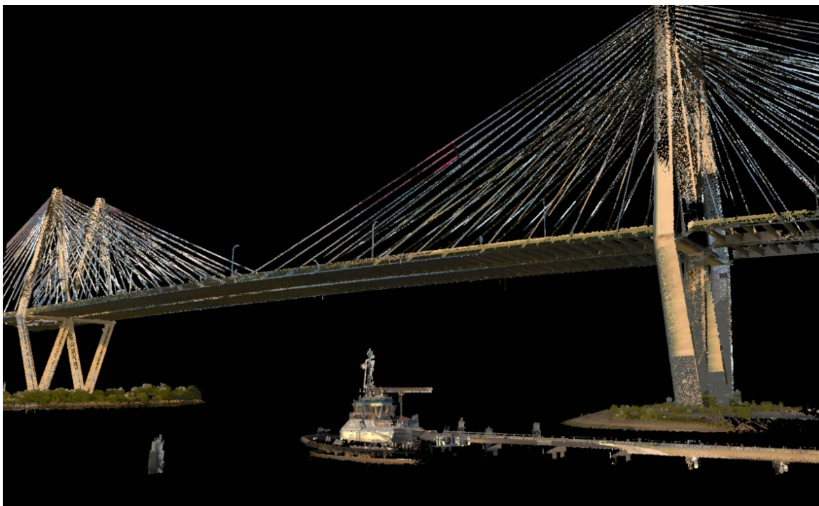
Fred Hartman Bridge, spanning the Houston Ship channel, laser scanned and colorized by David Evans & Associates for OPR-K375-KR-20.
